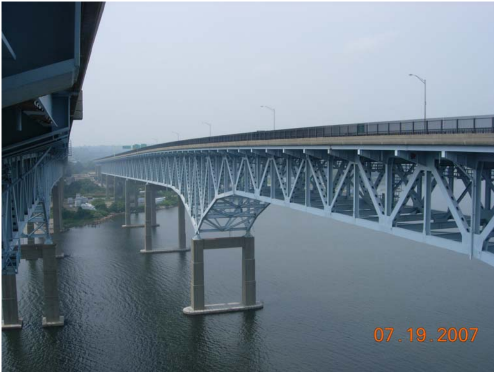
Figure 6. Goldstar Bridge over the Thames River in New London, Connecticut. Multiple solar powered nodes monitor strain and vibration at key locations on this structure.
