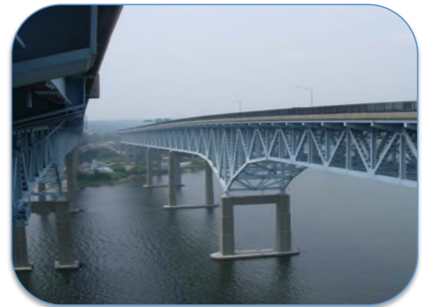
Figure 7. Goldstar Bridge in New Haven, CT
